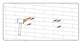
Figure 7-7 Knock the expansion tubes
